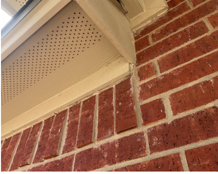
Expansion Joint Separation
