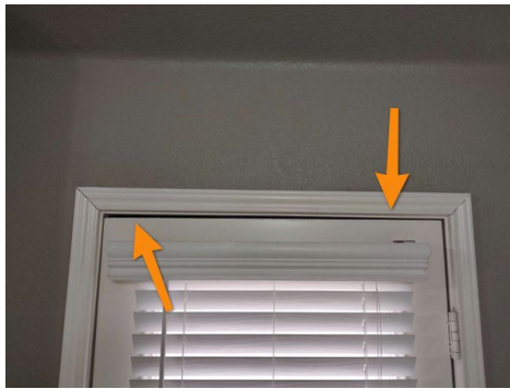
Doors Binding / Not Latching / Out of Square
