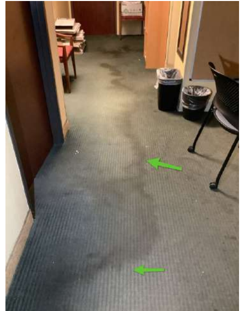
Employee area- entry
