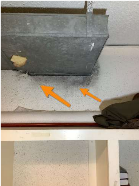
HVAC towel area#2 wall
