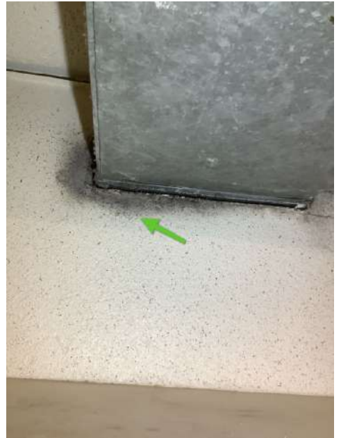
HVAC towel area wall -1
