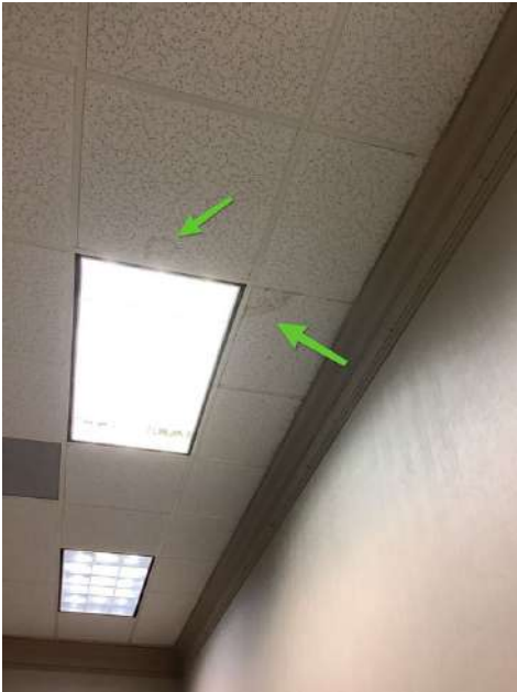
Warwick room - entry
