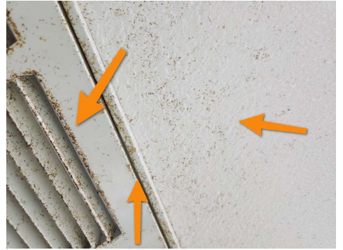
Downstairs kennel middle left side ceiling and Return
