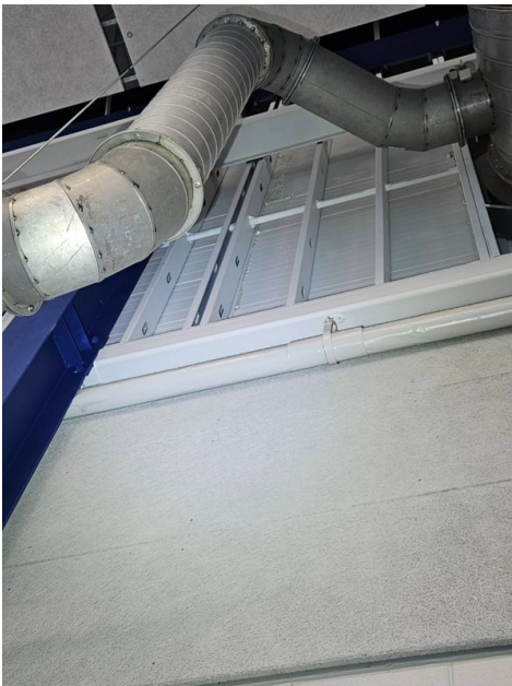
Left side of back wall above exit
