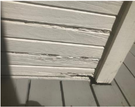
Exterior Distress: Rotted siding Unit 220, 224, 222, 2nd floor laundry, 102
