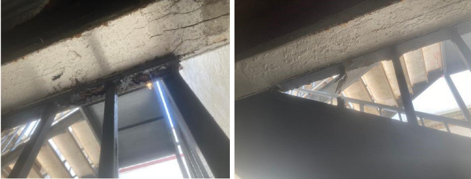
Exterior Distress: Significant Corrosion to Stair Railing East Stair
