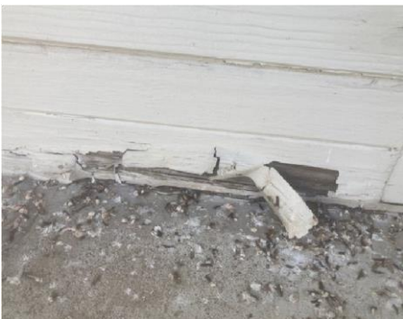
Exterior Distress: Rotted Trim Unit 207, 209, 210
