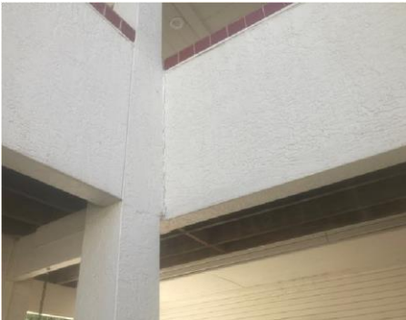
Exterior Distress: Stucco Cracks
