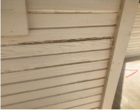
Exterior Distress: Rotted siding Unit 220, 224, 222, 2nd floor laundry, 102
