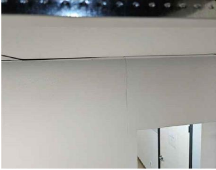
Wall below 2nd story addition
