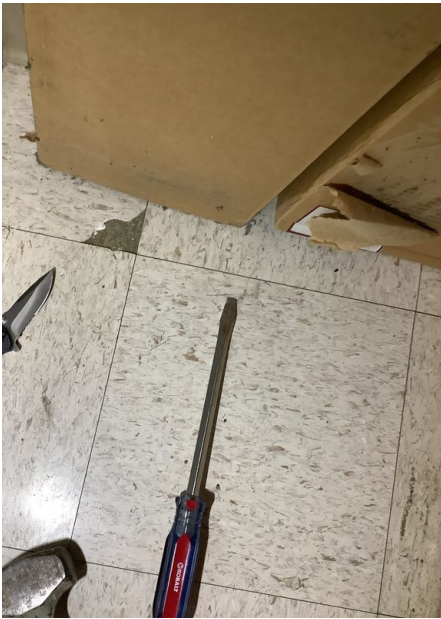
Tan floor tile & yellow mastic
