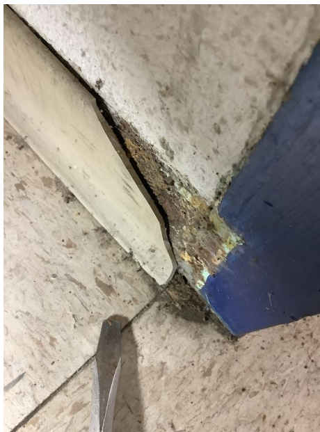
Tan cove base with mastic
