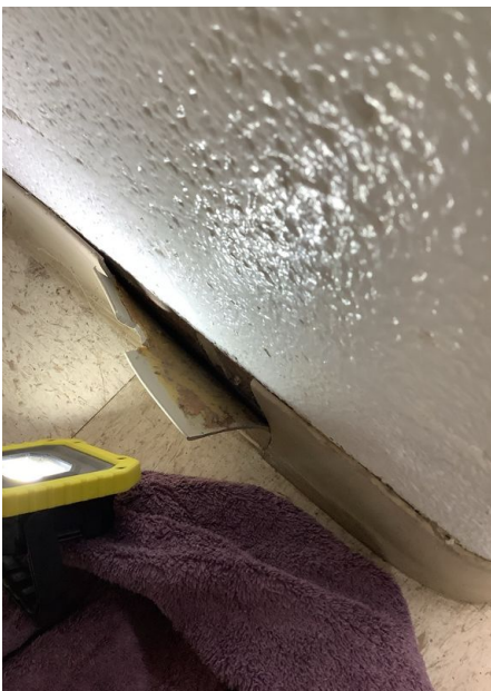
Tan cove base with mastic
