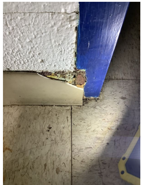
Tan cove base with mastic
