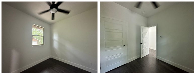
Interior Wall Finishes: Sheet Rock
