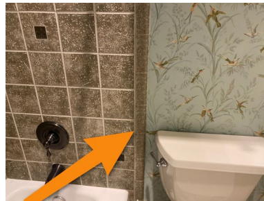
Downstairs Front Right Bathroom
