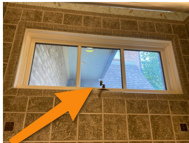
Downstairs Front Right Bathroom
