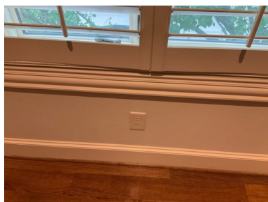
Upstairs Family Room
