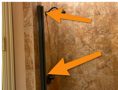
Upstairs Back Left Bathroom
