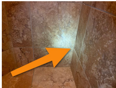
Upstairs Back Left Bathroom
