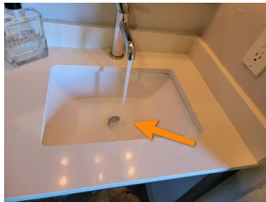
Downstairs Back Right Bathroom
