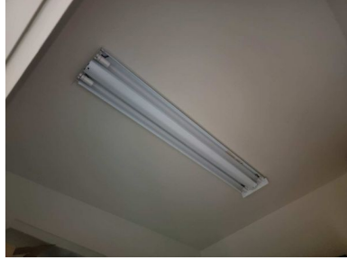
Upstairs Back Right Bedroom Closet
