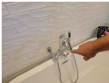
Downstairs Back Right Bathroom
