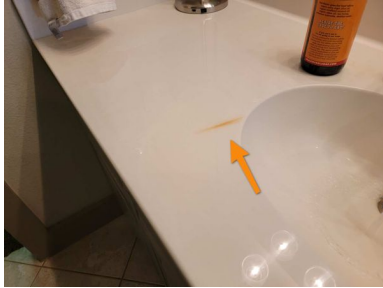
Upstairs Front Right Bathroom
